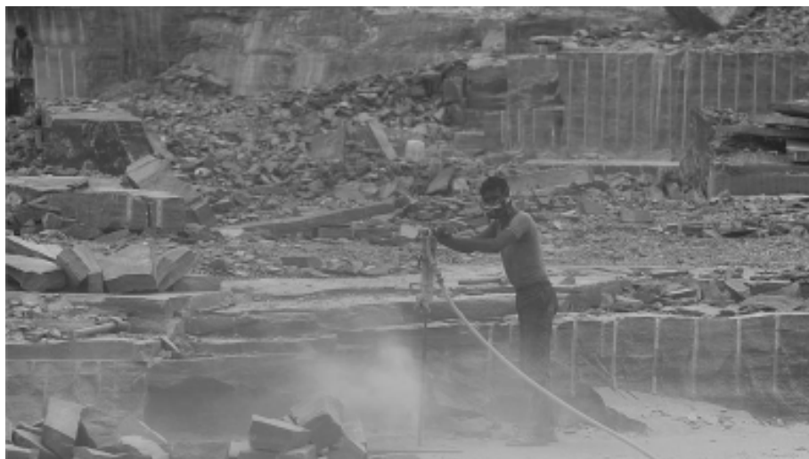
Figure 1 respirable dust generation during pneumatic drilling operation in Open cast mine
